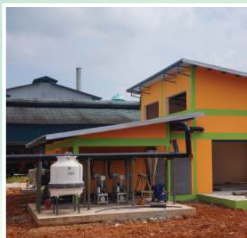
Capacity of wastewater 225 m 3 /day, COD 100,235 mg/l, Biogas Production 10,000-17,000 m 3 /day with Power Generation 2 MW, Palm Oil Mill
