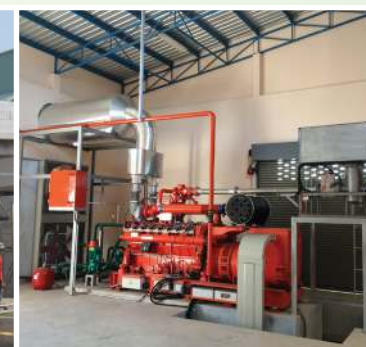
Gas Engine Generator, Palm Oil Mill
