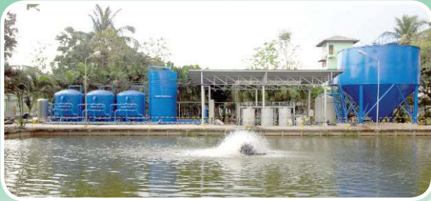
Water Recycle Plant 50 m³/hr, Food Processing Factory
