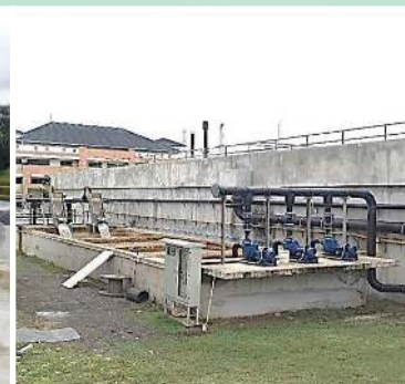
Capacity of wastewater 4,000 m 3 /day, COD 2,500 mg/l, Biogas Production 2,400 m 3 /day, Tuna Processing Factory
