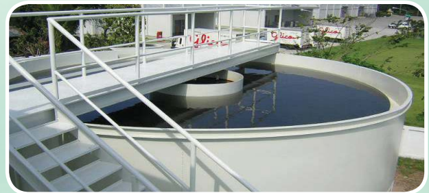
Wastewater Treatment Plant 1,200 m³/day, Electronics Factory
