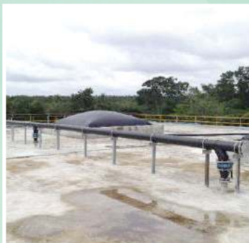
Capacity of wastewater 4,000 m 3 /day, COD 2,500 mg/l, Biogas Production 2,400 m 3 /day, Tuna Processing Factory
