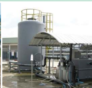
Capacity of wastewater 2,500 m 3 /day, COD 3,000 mg/l, Biogas Production 2,200 m 3 /day, Frozen Foods Factory
