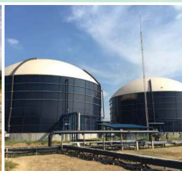
Capacity of wastewater 225 m 3 /day, COD 100,235 mg/l, Biogas Production 10,000-17,000 m 3 /day with Power Generation 2 MW, Palm Oil Mill
