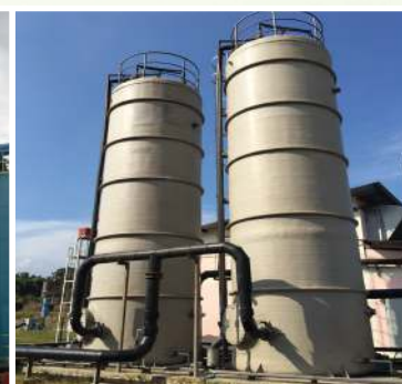
Biogas Upgrading and H 2 S Bio-Scrubber System, Palm Oil Mill
