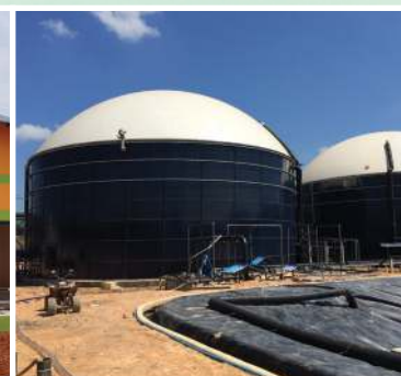
Capacity of wastewater 225 m 3 /day, COD 100,235 mg/l, Biogas Production 10,000-17,000 m 3 /day with Power Generation 2 MW, Palm Oil Mill
