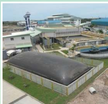
Capacity of wastewater 2,500 m 3 /day, COD 3,000 mg/l, Biogas Production 2,200 m 3 /day, Frozen Foods Factory
