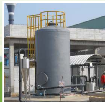
Biogas Upgrading and H 2 S Bio-Scrubber System, Frozen Foods Factory
