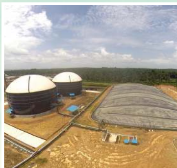
Capacity of wastewater 225 m 3 /day, COD 100,235 mg/l, Biogas Production 10,000-17,000 m 3 /day with Power Generation 2 MW, Palm Oil Mill
