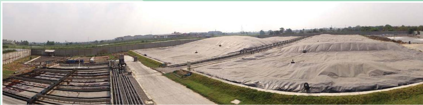
Capacity of wastewater 2,000 m 3 /day, COD 6,500 mg/l, Biogas Production 4,000 m 3 /day, Coconut Milk Processing Factory
