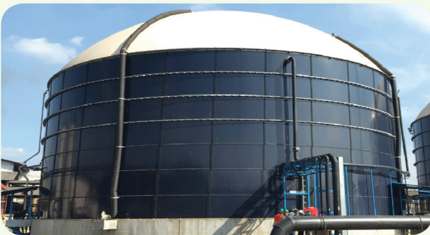
GFS Bolted Tank & Double Membrane Gas Storage
