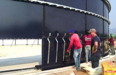
Tank Diameter 28.15 m. Tank Height 11.08 m. Tank Capacity 6,584 m³ Quantity 3 Tanks Gas Mixing System 18.5 kW 3 Units/Tank
