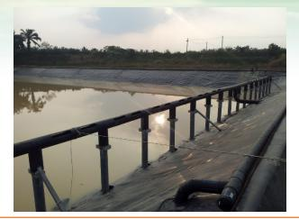
Biogas Collecting Pipes, HDPE Lining Sheet
